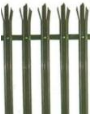
No splay - cut spikes that could trap fingers and leave someone hanging.
